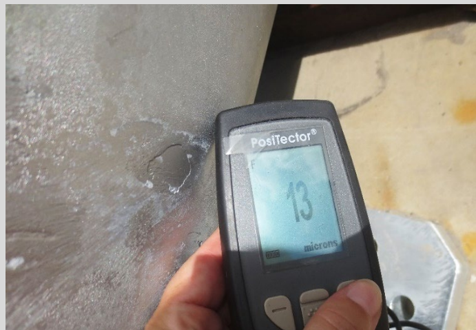
Figure 11.2.4 – Coating thickness reading on zinc spray
