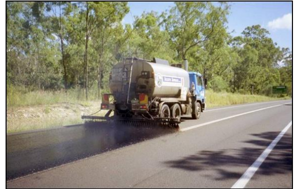
A bitumen sprayer in action
