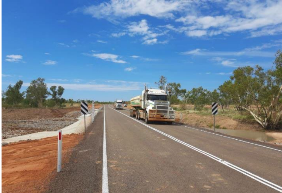
Aramac Torrens Creek Road, Aramac
