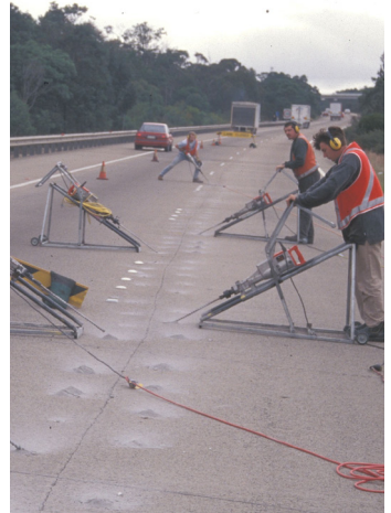
Cross stitching concrete surface repair
