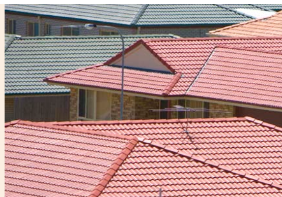
Residential housing. Source: TMR
