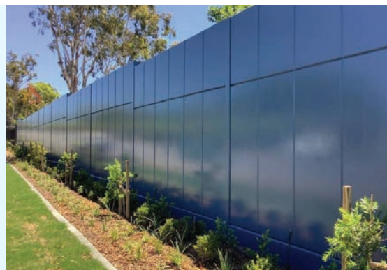
Noise barrier. Source: TMR
