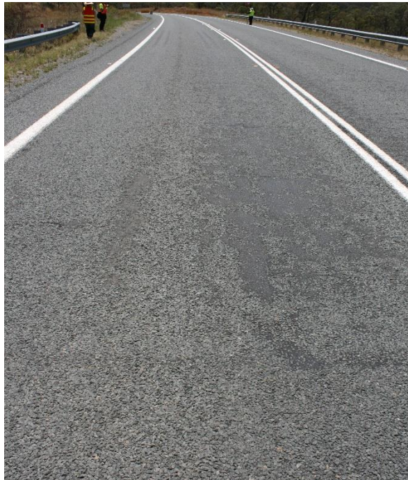
Figure 2 – Stripping of a sprayed seal
