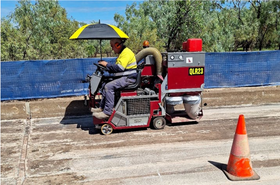
Figure 10.6.1(c) – Bobcat with a poly planer head with multi-row teeth
