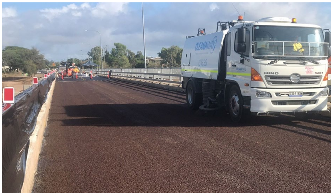
Figure 10.10(a) – A vacuum truck with side brushes removing loose aggregates
