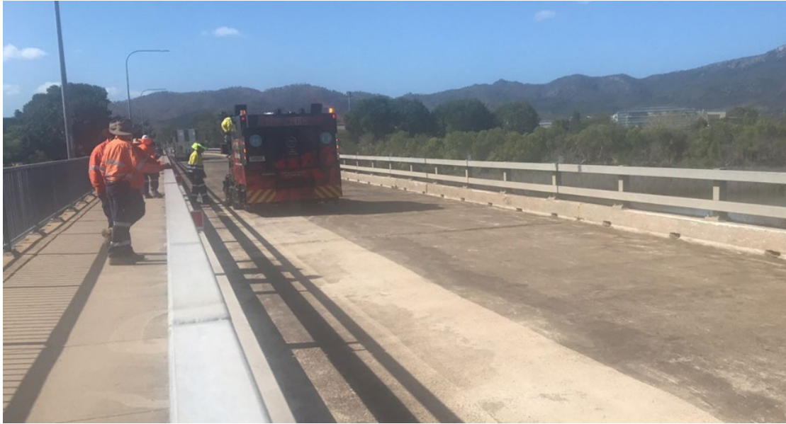
Figure 10.6.2(b) – Final cleaning and retexturing concrete bridge deck using a small shot-blasting machine
