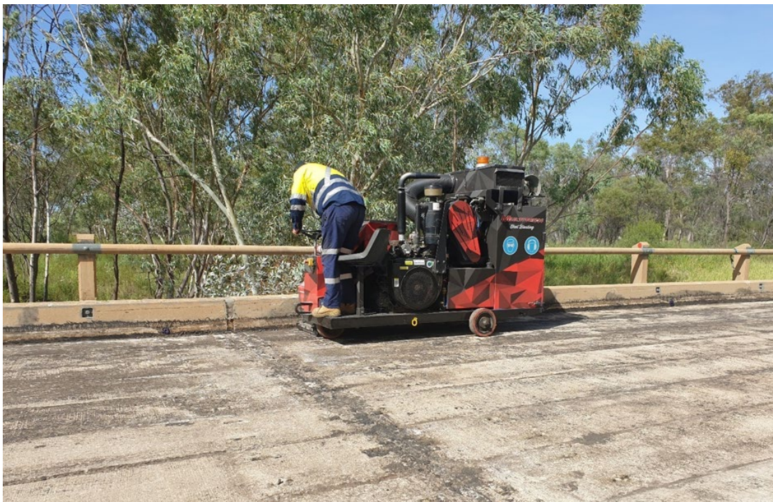
Figure 10.6.2(b) – Final cleaning and retexturing concrete bridge deck using a small shot-blasting machine
