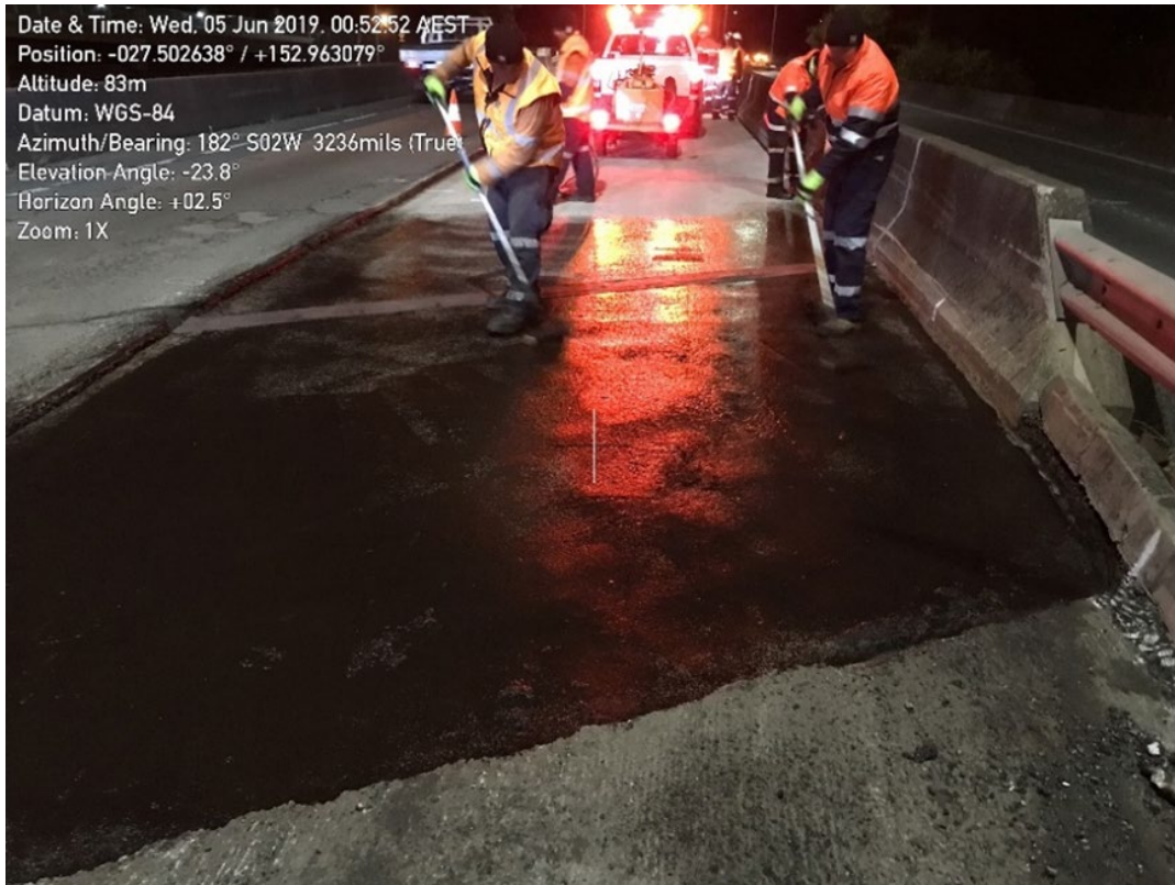
Figure 10.9(a) – Paint rollers used to spread and remove excess of concrete prime
