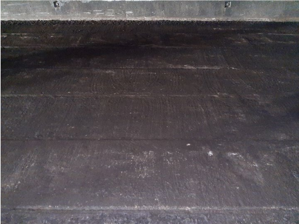
Figure 10.6.1(e) – Concrete bridge deck units after cleaning / sweeping
