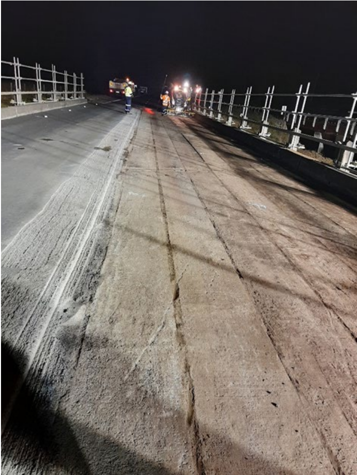
Figure 10.6.1(e) – Concrete bridge deck units after cleaning / sweeping
