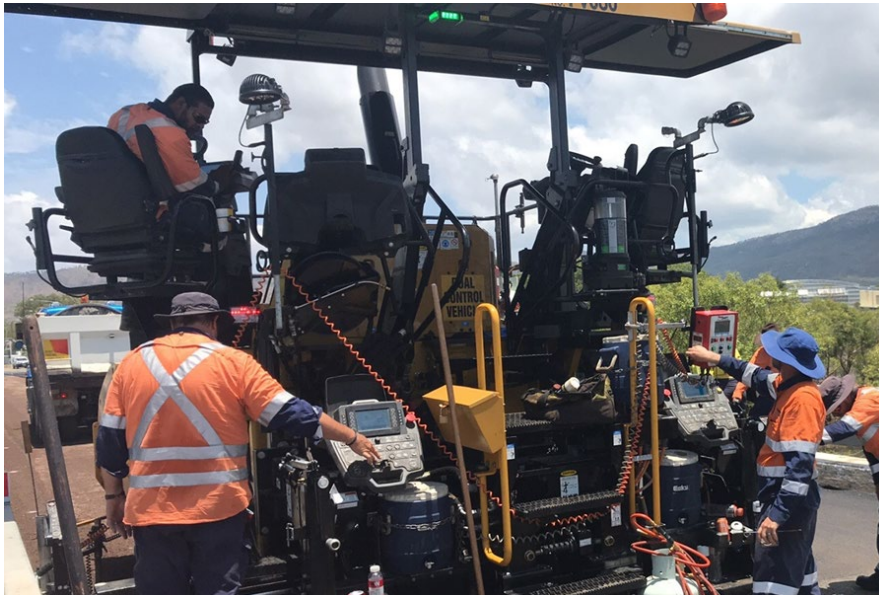
Figure 10.11(d) – Use of computerised asphalt grade level control (red panel) for improved asphalt DWS thickness precision
