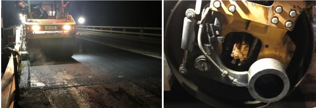
Figure 10.11(d) – Use of computerised asphalt grade level control (red panel) for improved asphalt DWS thickness precision
