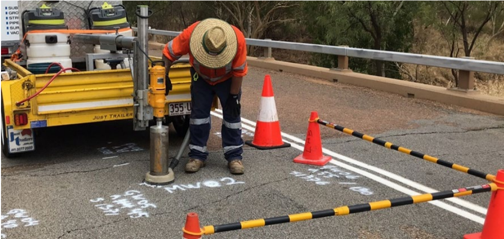
Figure A3 – DWS coring (to calibrate CPR depth scanning)
