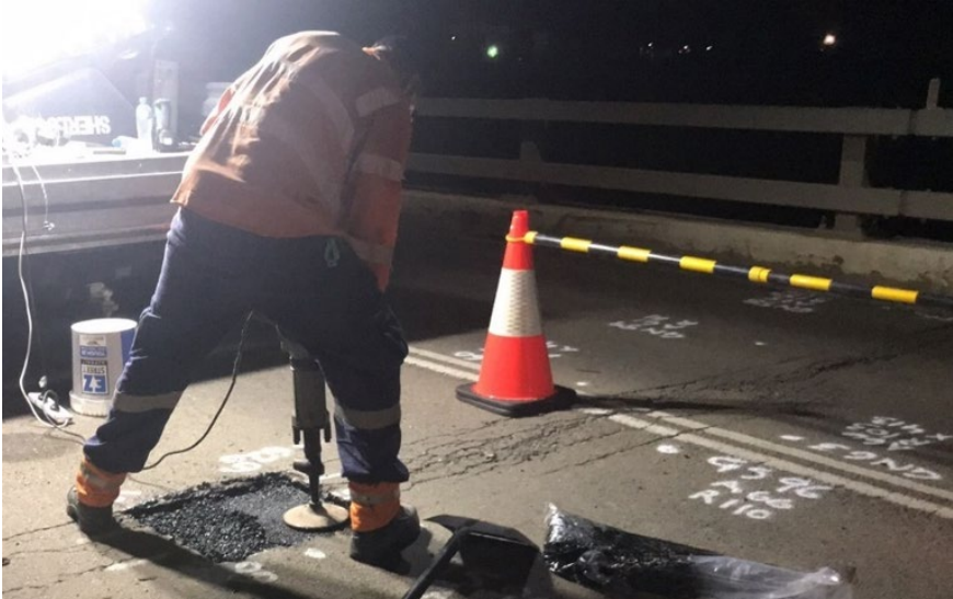
Figure A6 – Hot mix asphalt reinstatement
