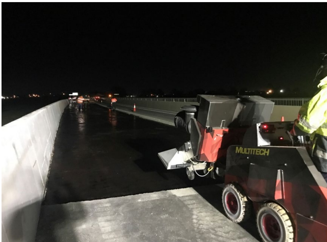
Figure 10.9(b) – Jet blower road heater used to accelerate concrete prime curing
