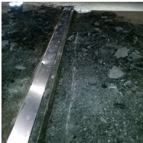
Figure 10.5 – Temporary metal cover plate to protect an expansion joint
