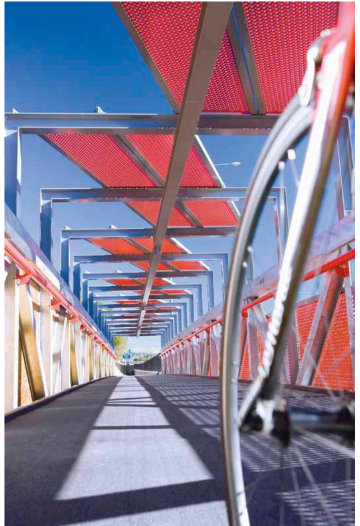
Veloway Cycleway linking Brisbane's CBD with the Gateway off-ramp at Eight Mile Plains
