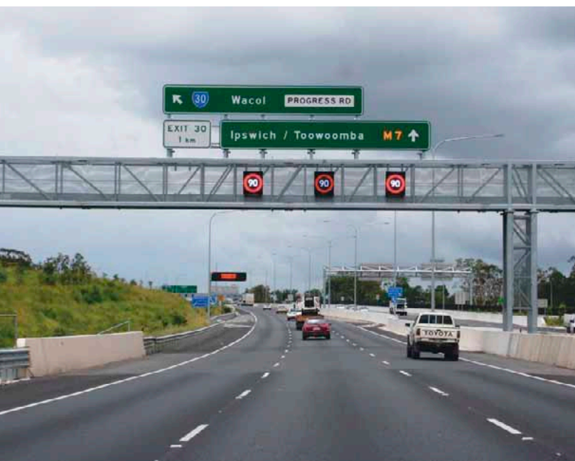
One of the many intelligent transport systems over the Ipswich Motorway
