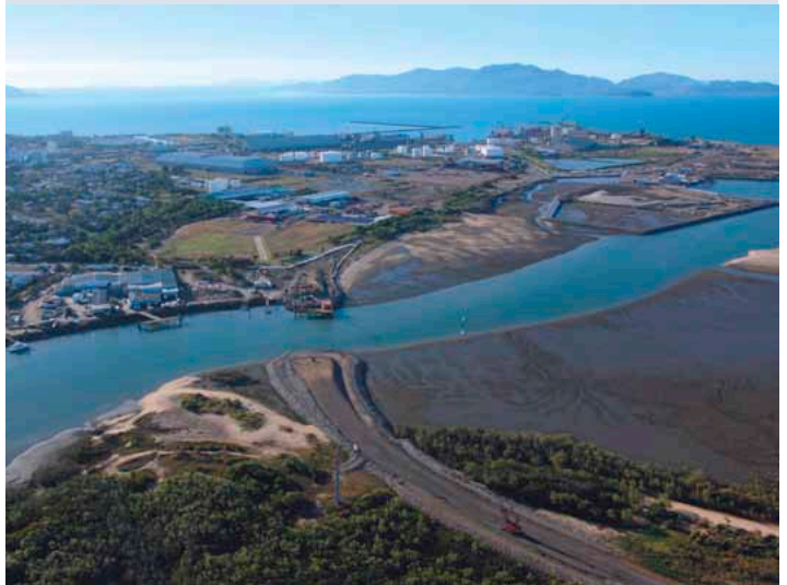
Aerial view showing construction of the Townsville Port Access Road
