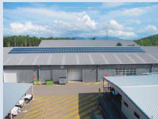
Solar panel project at the RoadTek Townsville Works Centre
