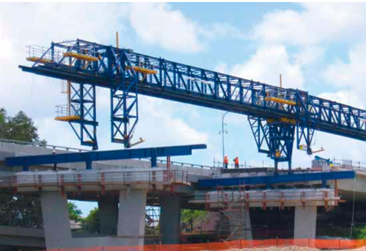
Left: This large truss can lift heavy frames and is powered by vegetable oil
