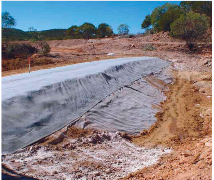
Improvement works at Federation Mine near Croydon
