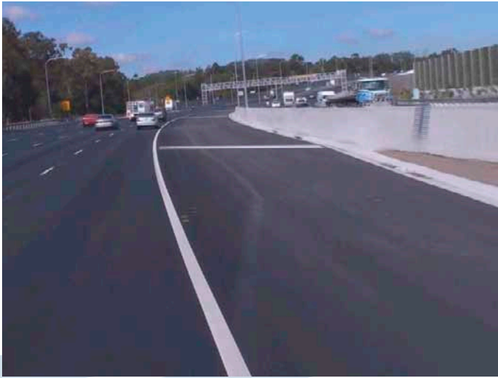
Road shoulder under the new guidelines
