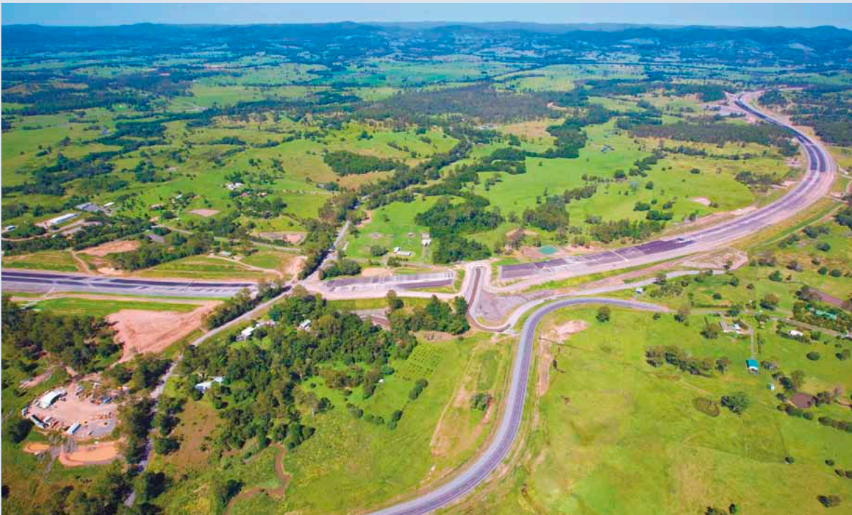
Aerial view of the Bruce Highway upgrade at Coles Creek Road
