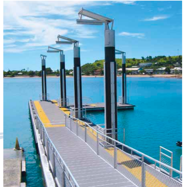
The new pontoon at Thursday Island
