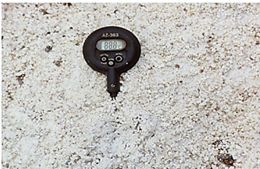
Figure 8.6.5.3 – Checking completion of slaking with temperature probe
