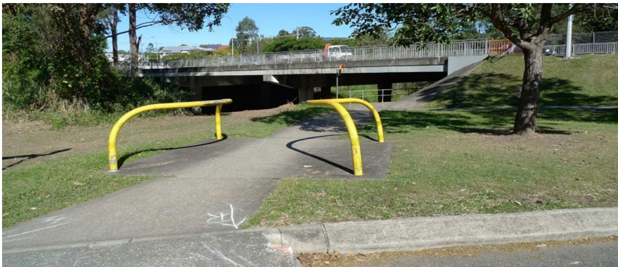
Figure C.3 – Redundant path terminal barrier
