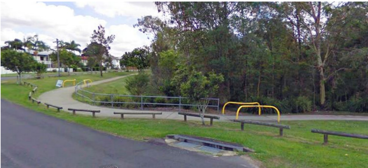
Figure C.2 – Excessive use of physical barriers to slow people riding bikes on approach to a blind corner
