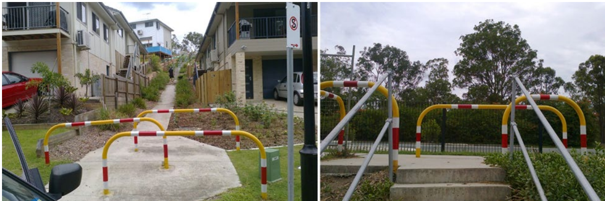
Figure C.5 – Redundant U-rail type barrier on a set of stairs
