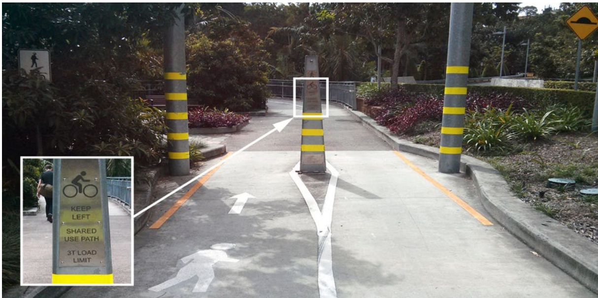
Figure C.13 – Examples of the use of bollards to protect an asset, with instructive text
