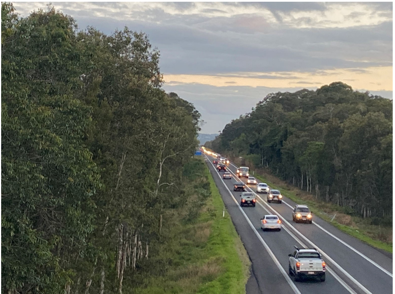
Image: TMR – Sunshine Motorway, south of Coolum.
