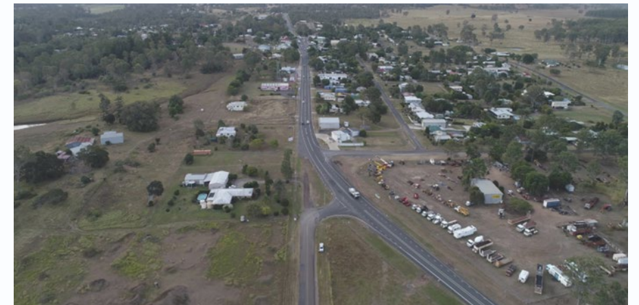
Existing Bruce Highway at Tiaro looking North
