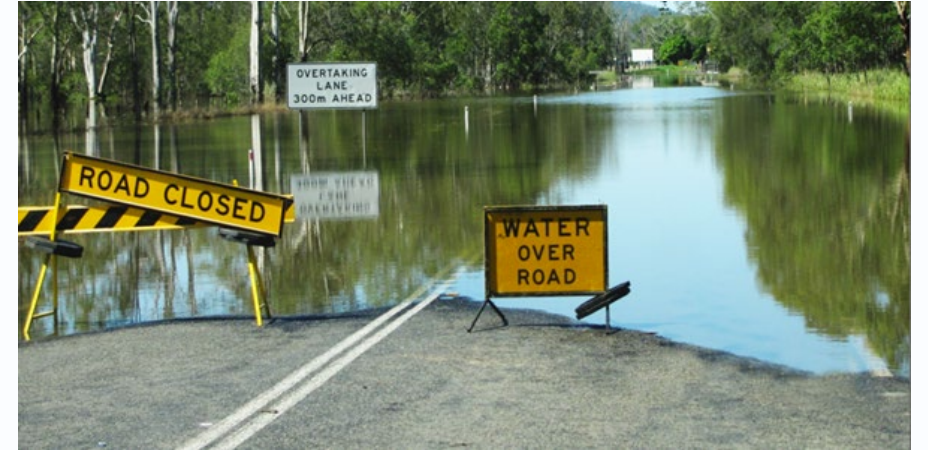
Existing Bruce Highway at Chinaman Creek North of Tiaro - Flooding Event
