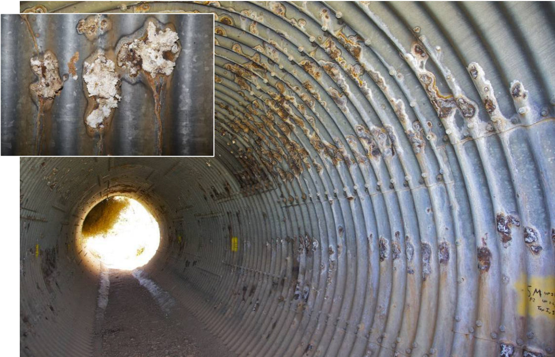
Figure 8 - A culvert exhibiting perforations due to corrosion to the upper portion of the culvert
