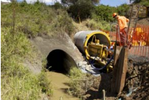
(a) thrust block and hydraulic rams
