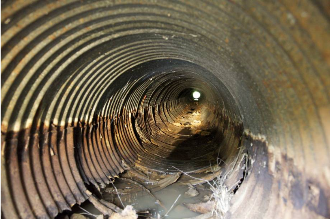
Figure 8 - A culvert exhibiting perforations due to corrosion to the upper portion of the culvert
